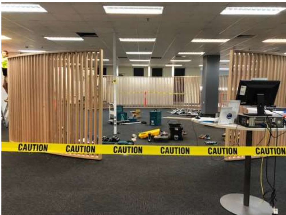
Elgar library mid-renovation
